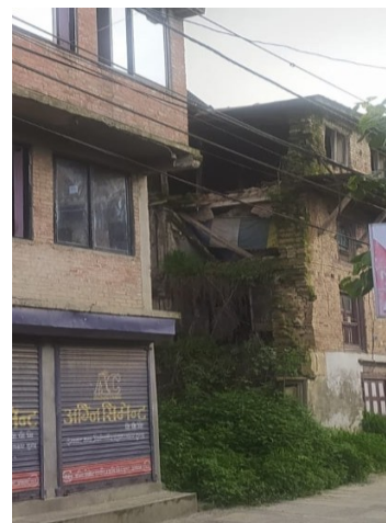
Figure 9 one section demolishes
